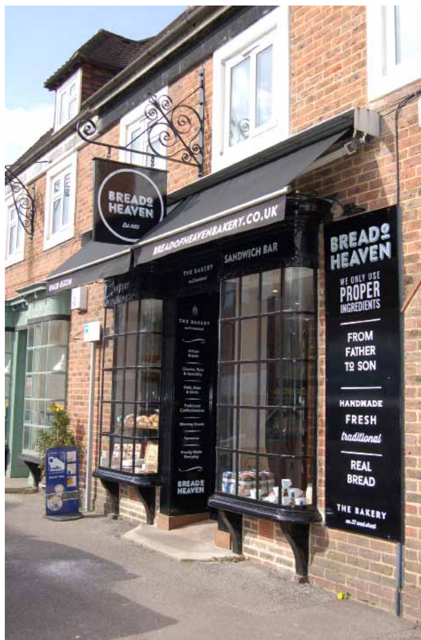
Figure 12. West Street, Haslemere: The incorporation of a retractable awning on this shopfront does not dominate over the overall frontage and allows for flexibility of use. The awning blends into the shopfront in terms of colour and is of a traditional style that complements and enhances the shopfront.
