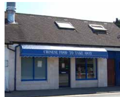
Figure 9. Ewhurst Road, Cranleigh: An example of marble shopfront which is not considered best practice.
